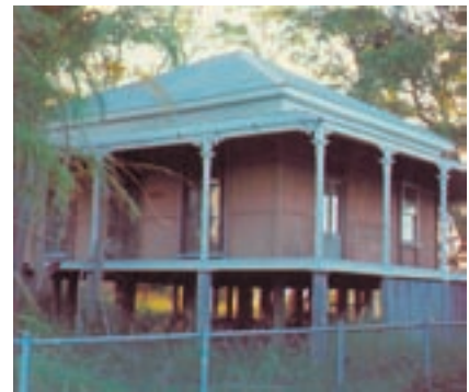
Early housing used verandahs to protect cladding
