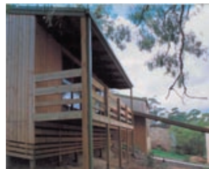
Preservative treated pine cladding - vertical fixing
