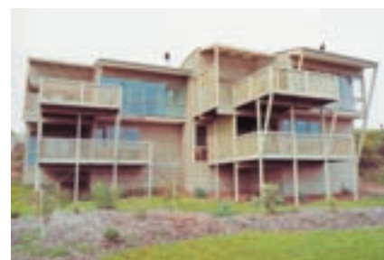
Sawn weatherboards finished with semi-transparent stain on multi-residential units
