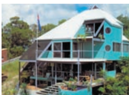
Versatile plywood cladding - grooved and sawn textured finish
