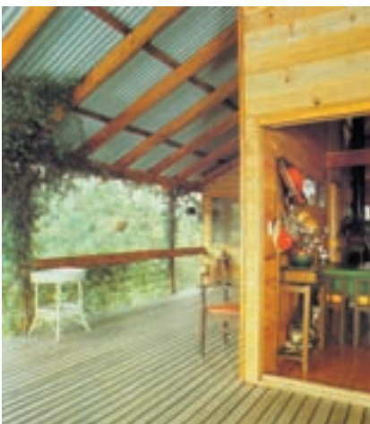
Verandah roofs or eaves overhang provides good protection to timber cladding
