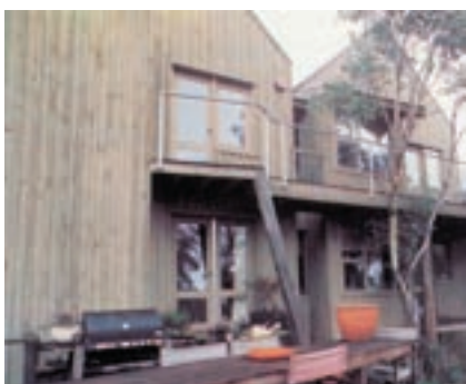
Semi-transparent stained board and batten cladding
