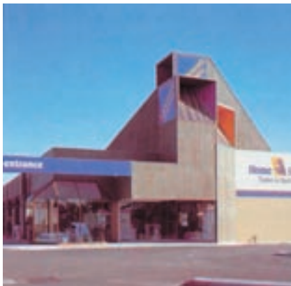
Plywood cladding can also act as structural shearwalls
