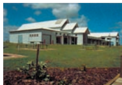
Opaque finished hardwood cladding protects sea-front tourist complex
