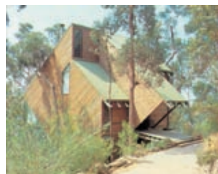
Preservative treated pine cladding reflects roof shapes
