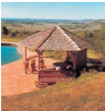
Poolside shelter roofed with shingles
